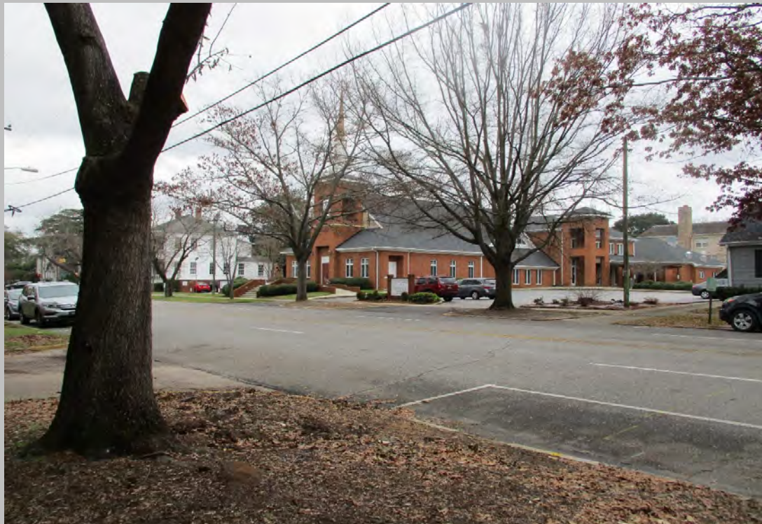
View of the southern adjacent Korean Presbyterian Church
