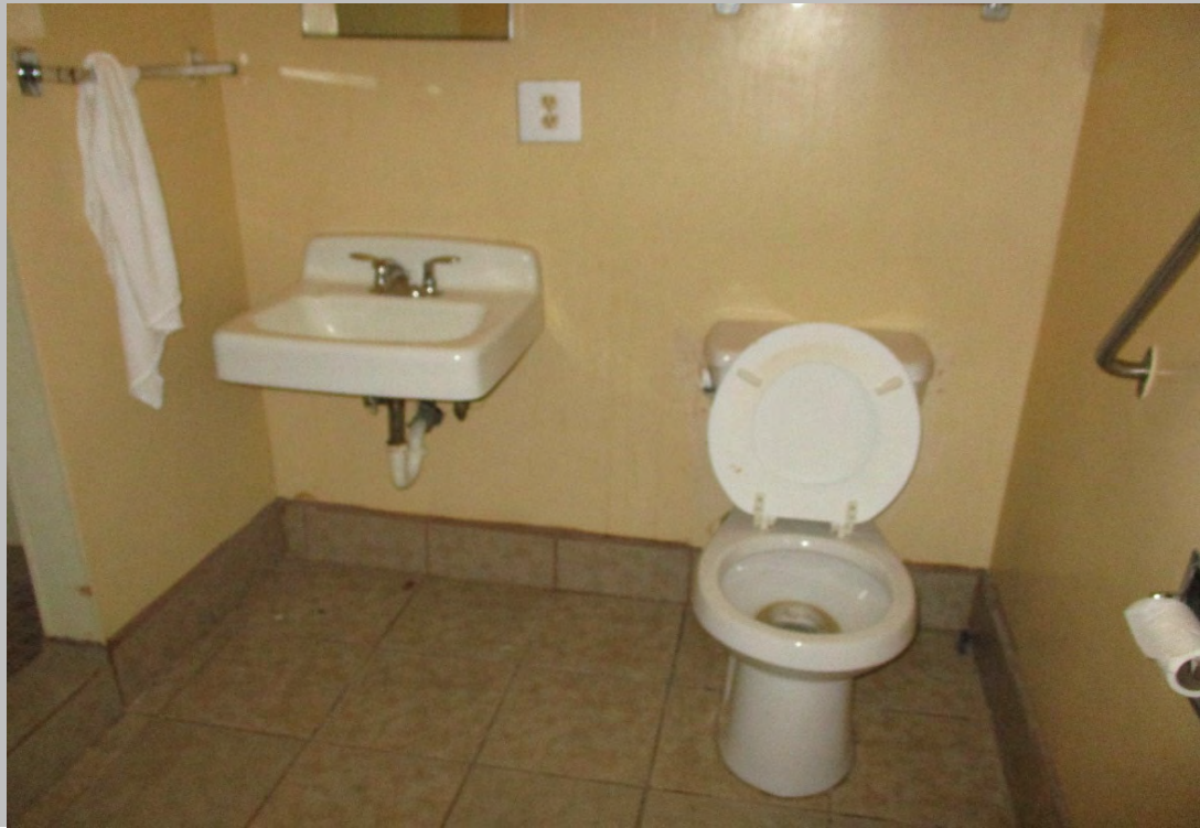
View of a typical residential unit bathroom
