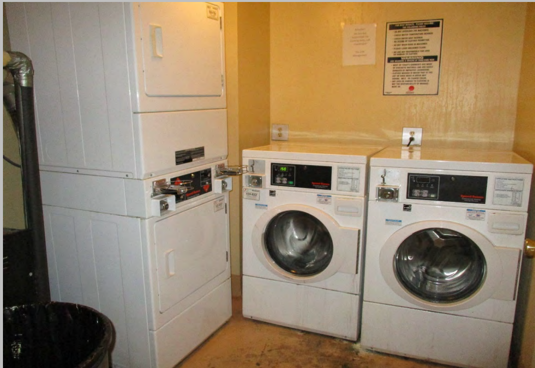
View of the laundry facilities
