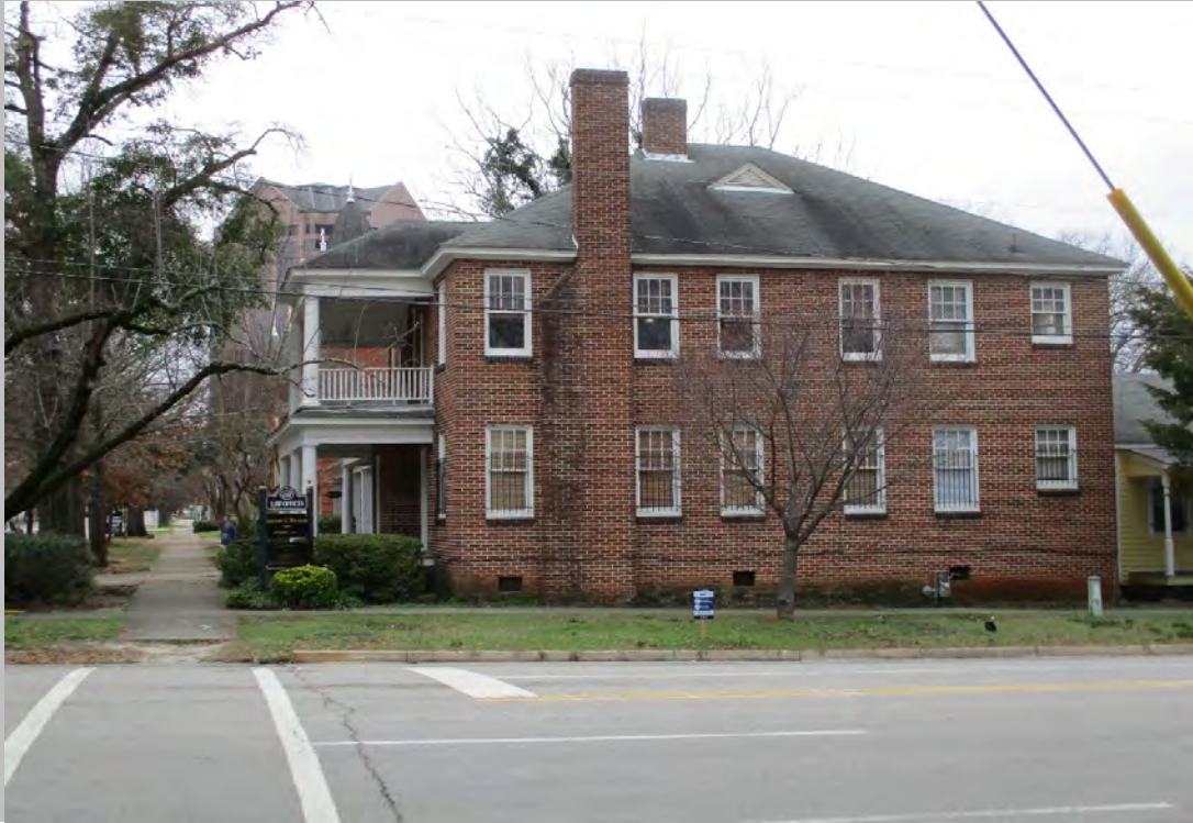
View of the western adjacent Law Offices
