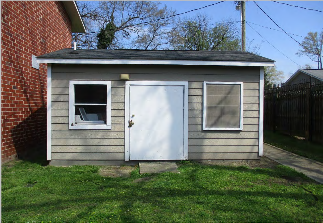
View of the exterior of the on-site laundry structure
