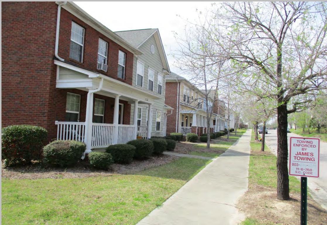
View of the southern adjacent single-family residential homes
