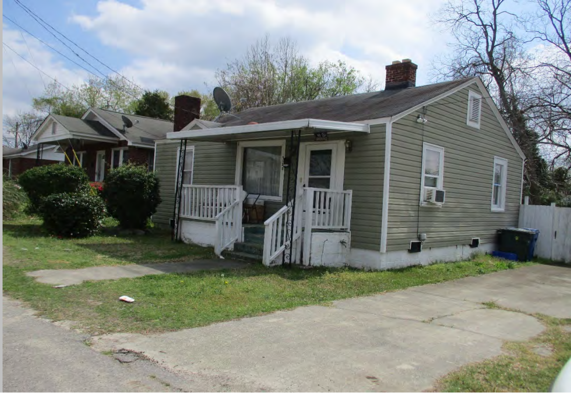
View of the northern adjacent single-family residential homes
