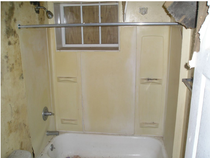
Photo 9 – Typical view of tub surround.
