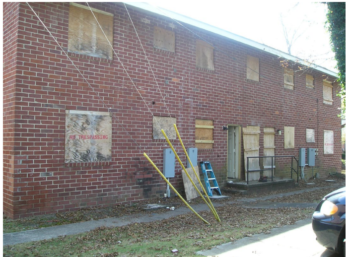
Photo 4 – Typical view of rear of apartments.
