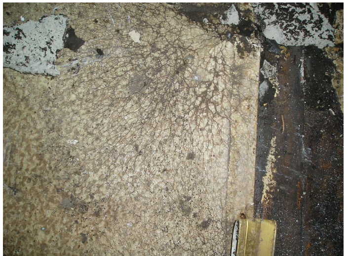
Photo 6 – Typical view of Kitchen flooring.
