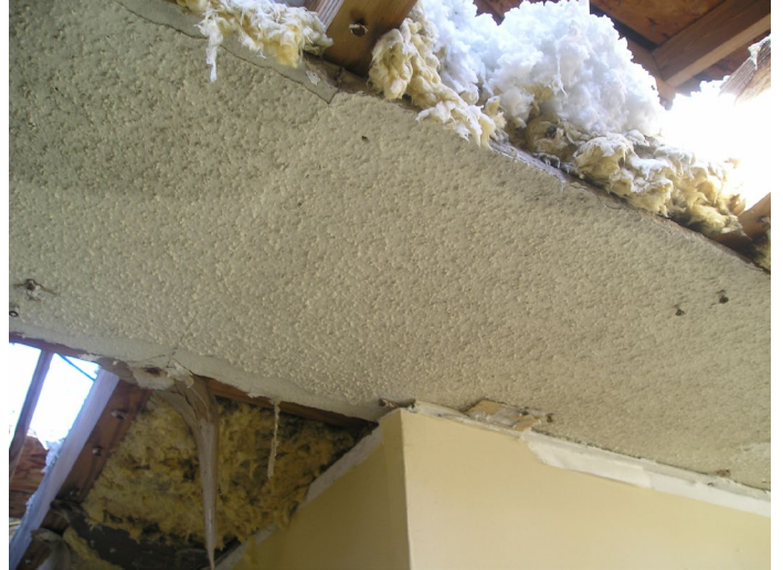
Photo 14 – Upstairs ceiling texture.
