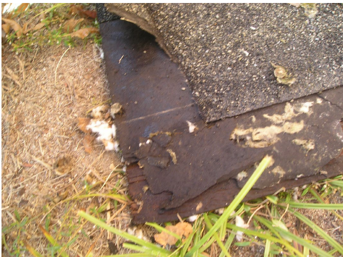
Photo 17 – Roof shingles and felt.
