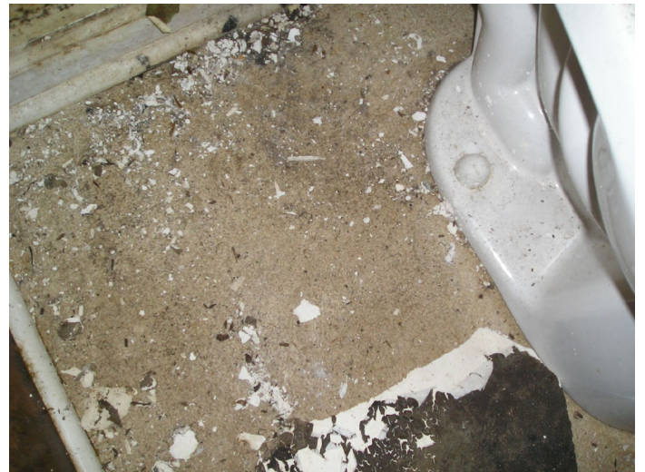
Photo 10 – Typical view of vinyl bathroom flooring.
