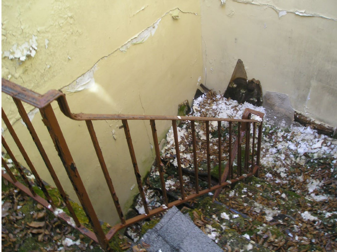
Photo 13 – Entry stair well with plaster and stair tread.
