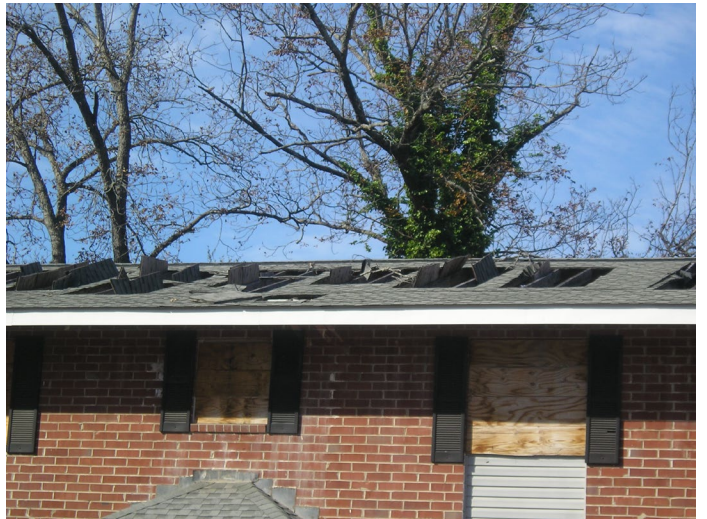
Photo 2 – Holes cut through roofs prior to survey.
