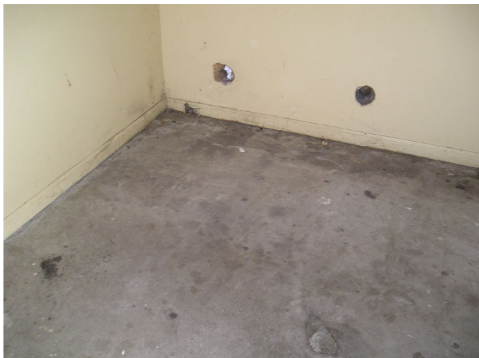
Photo 19 – Laundry shed drywall with concrete slab.
