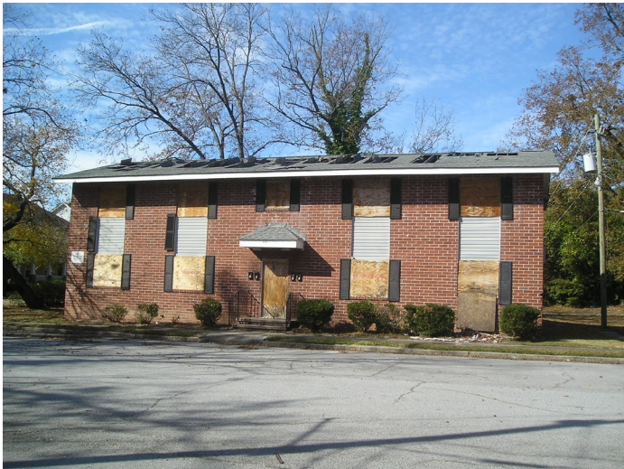
Photo 1 – Front view Columbia Apartments.
