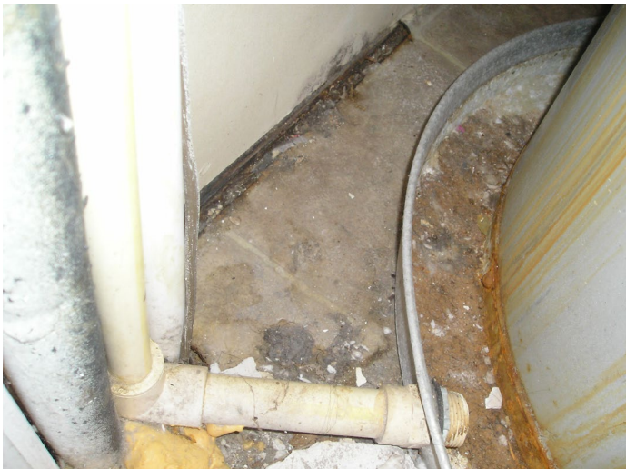
Photo 15 – Typical view of vinyl flooring in HVAC closets.
