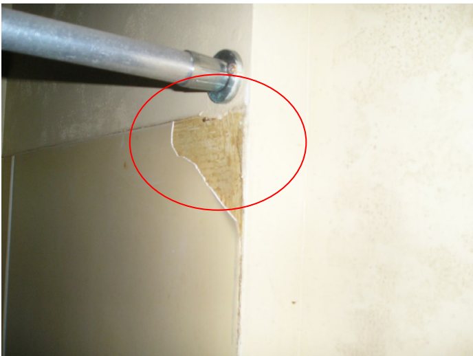
Photo 11 – Typical view of tub surround mastic.
